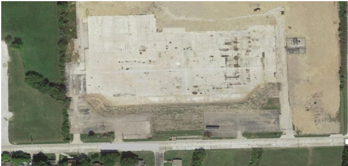
Figure 1: Former manufacturing site in Danville, IL
